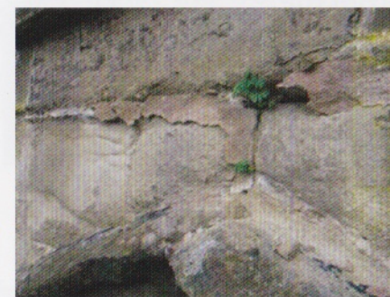
Examples from the exterior of St Anne's Chapel showing open joints and decayed stone allowing water ingress.
