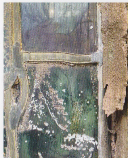
Examples from the exterior of St Anne's Chapel showing open joints and decayed stone allowing water ingress.
