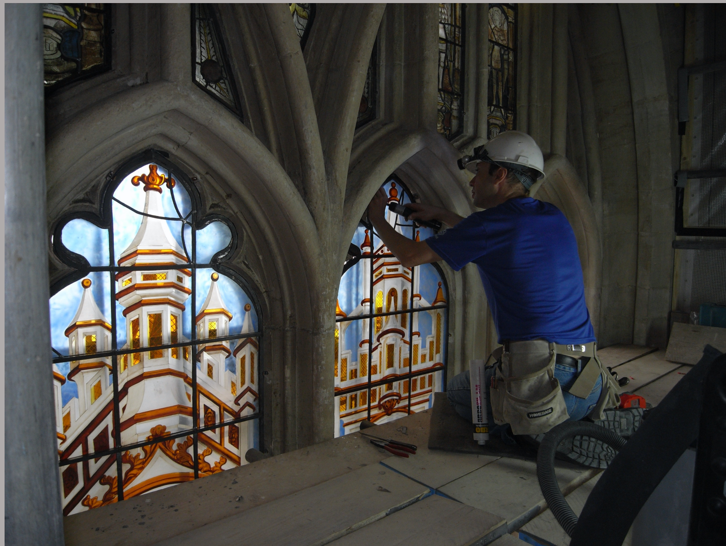
New College Chapel nV: outer glazing matched to patterns of the ferramenta – simple and cheap to make
